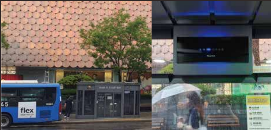
- Gangnam-gu Office Fine Dust Free Shelter
