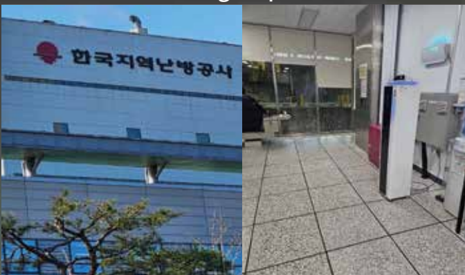
- Korea District Heating Corporation
